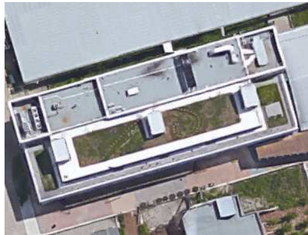
Fig. 3: Evergreen Brick Works Green Roof (photo: Google)
