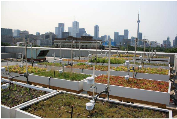
Fig. 2: GRIT Lab Roof (photo: GRIT Lab)
